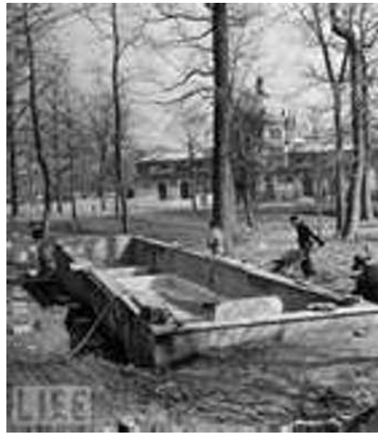
Platypus pool being built
